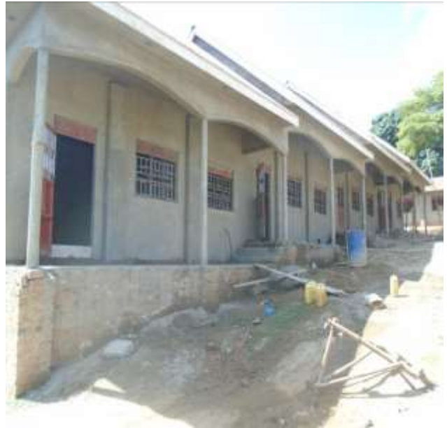
After roofing and plastering
