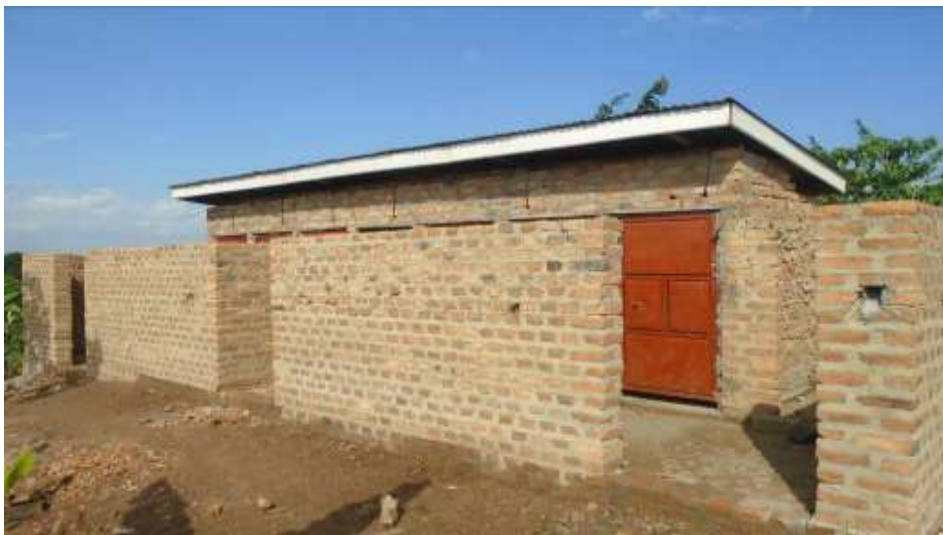
The pit latrine after roofing and shuttering
